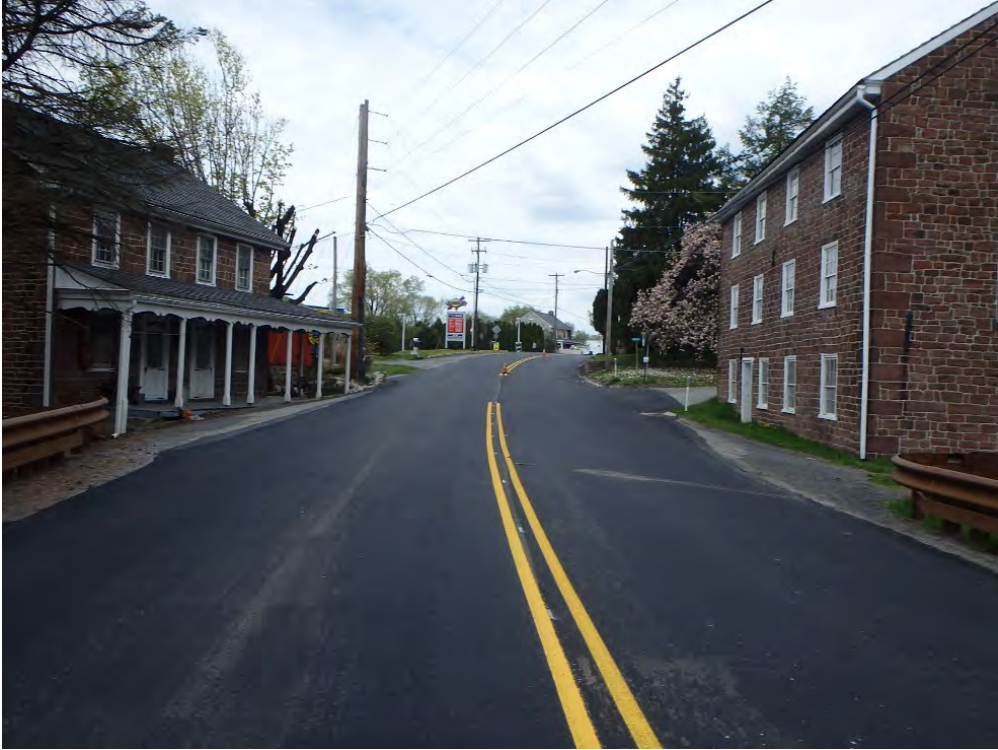
Photo 5: SR 625 with the Bowmansville Roller Mill at the right of photo and the miller's house to the left in photo.
