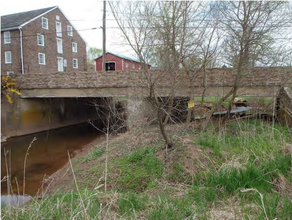
Photo 4: Bowmansville Bridge and mills.
