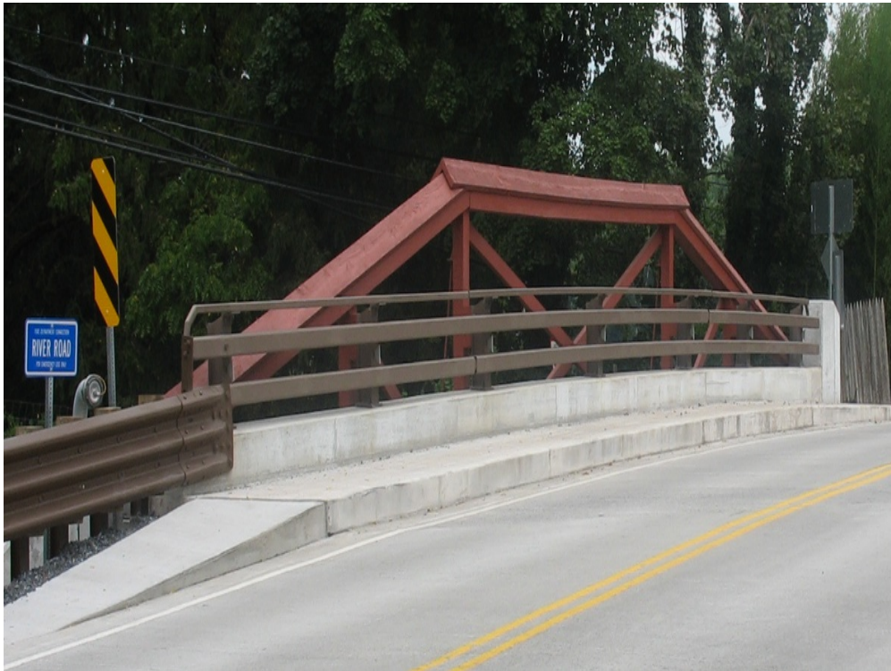
Photo 6: Painted guide rail.
