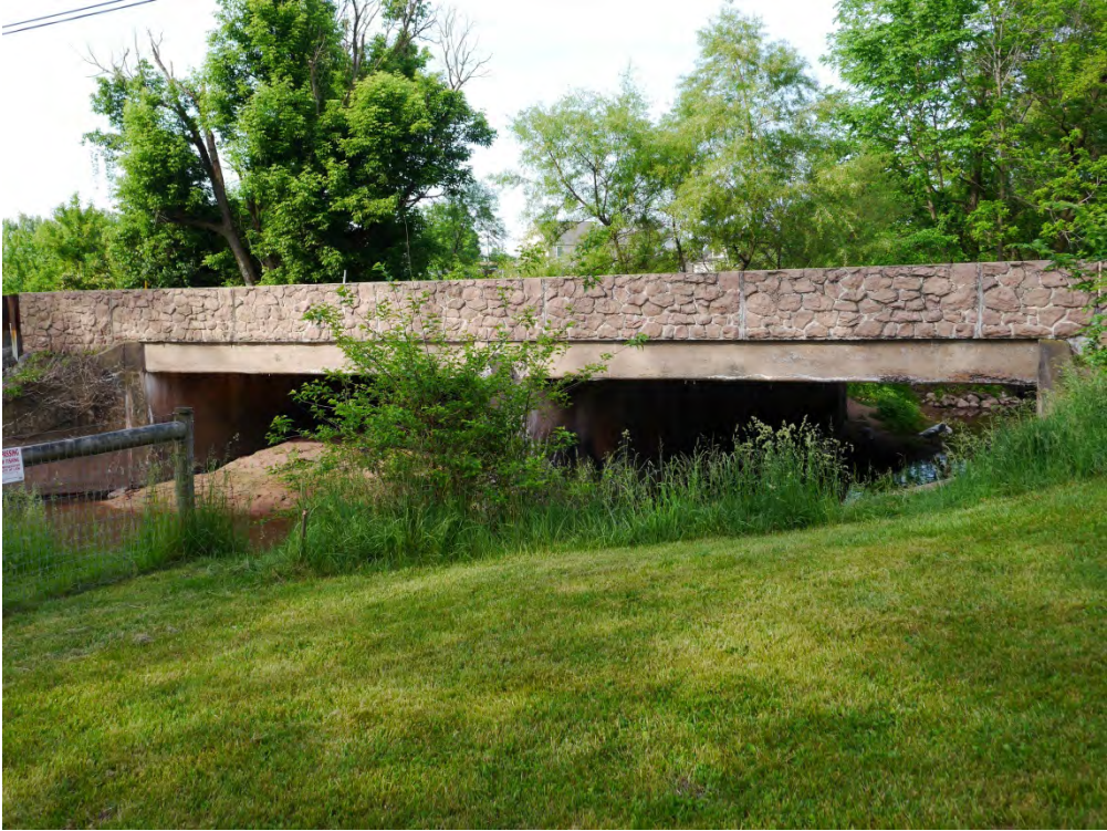
Photo 2: Bowmansville Bridge on SR 625 in Brecknock Township, Lancaster County. The bridge form liner was designed to mimic the stone in the roller mill adjacent to the bridge.
