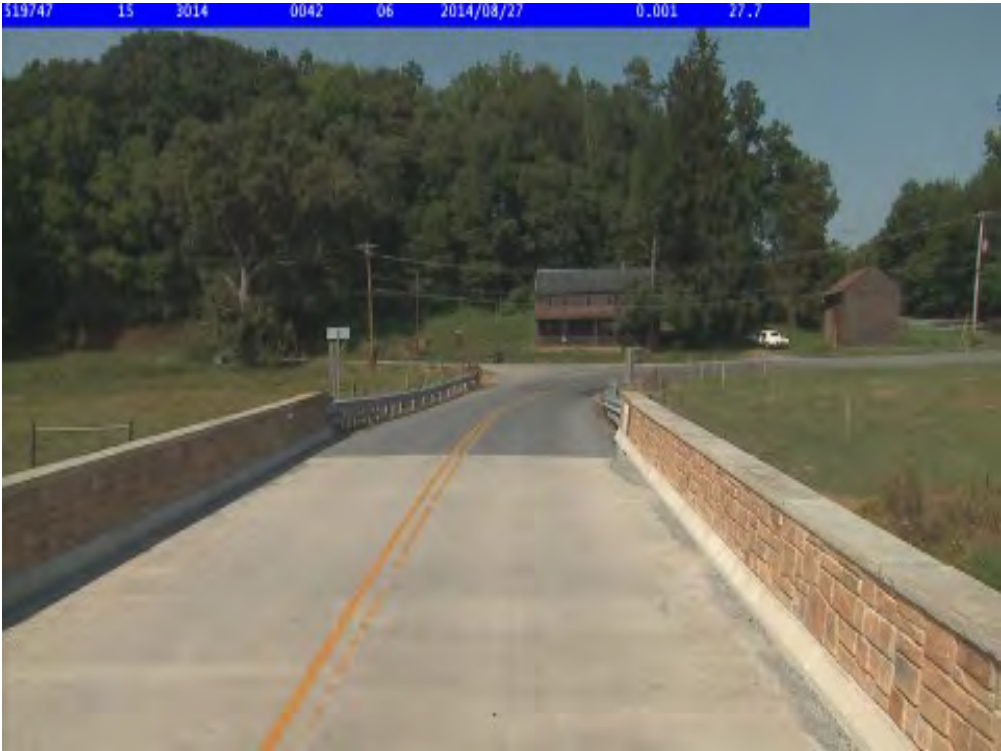
Photo 1: SR 3014 Lees Bridge Road, West Nottingham Township, Chester County. The Original 1915 bridge had a similar stone parapet with concrete coping.
